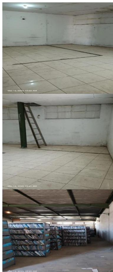
Figure 1. Medical Record Storage Building
